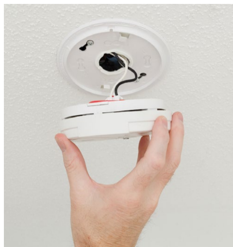
Regular maintenance should be viewed as an investment.
