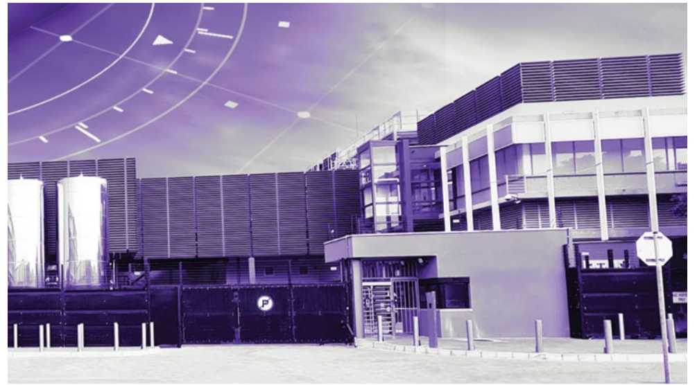
This expansion shows the data centre giant adding three new state-of-the-art halls in new areas on the campus and adds another 6MW of IT load.
