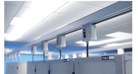
Busway power distribution provides an innovative, customisable power distribution and monitoring solution that meets each customer's critical requirements.
