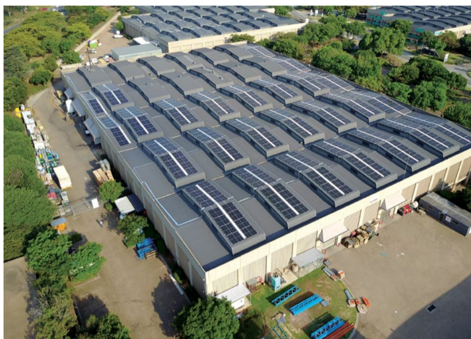
LESCO Manufacturing's factory has been fitted with a solar photovoltaic system to reduce the company's reliance on Eskom, while also being more environmentally conscious.
