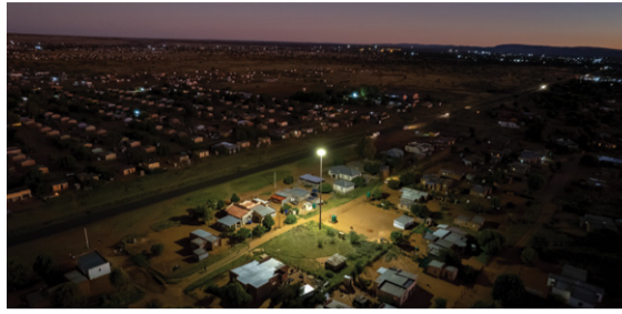
The existing HID 400W HPS highmast lighting was replaced with the newly launched OMNISTAR-ECO floodlight.
