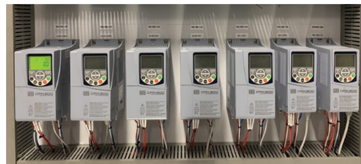
A range of WEG Variable Speed Drives that can prevent equipment from tripping out during load shedding.
