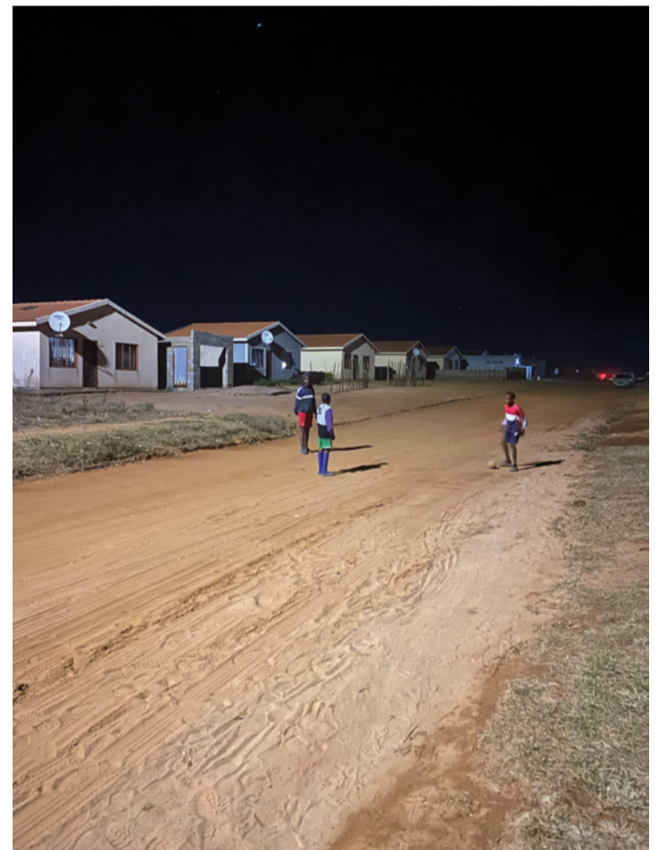
The solar lighting highmast solution increases the safety and well-being for the community.
