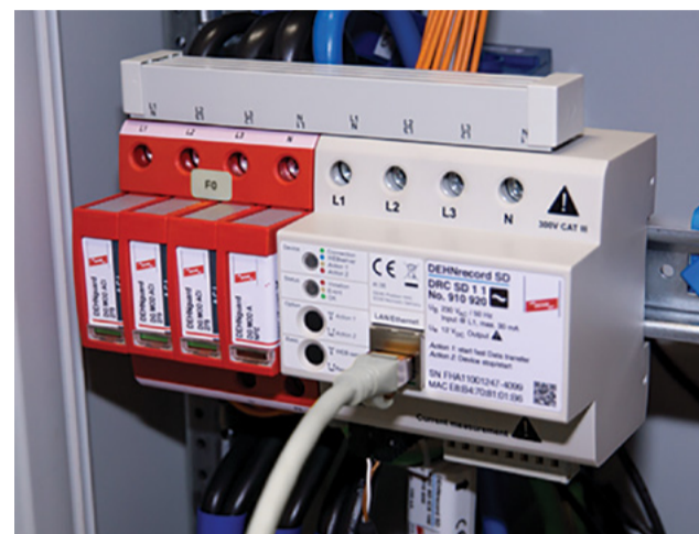
Example of a smart PQ measurement device capable of measuring surge and lightning impulse.
