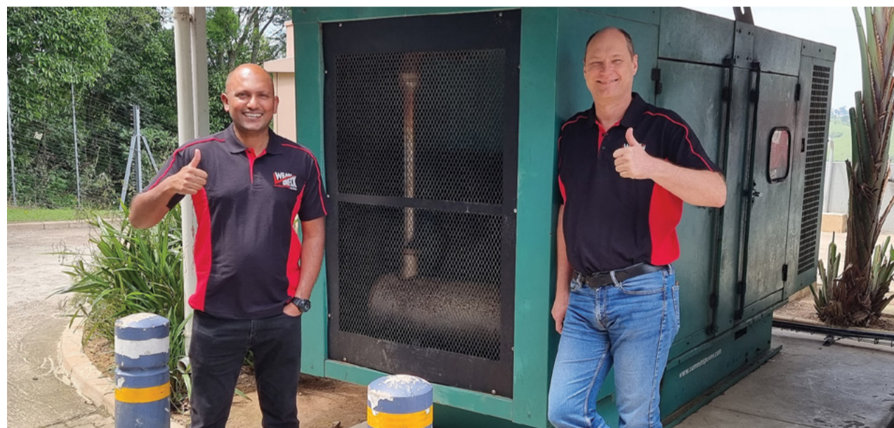
Thumbs up to a seamless power solution - WearCheck's major laboratories in South Africa and beyond are equipped with generators to ensure uninterrupted operation during electricity power outages. The company's laboratory manager, Meshach Govender (left), and managing director, Neil Robinson, are seen here with the generator at WearCheck's Durban, Westville, laboratory.
