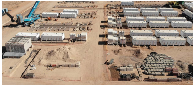
BESS Installation, Scatec Kenhardt facilities.
