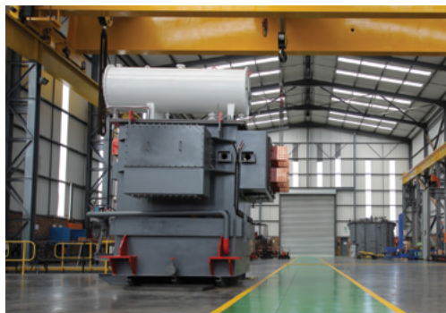
The Zest WEG manufacturing facility for large transformers in Heidelberg.
