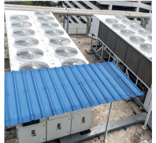
The WEG IE5 electronically commutated motors are well suited for fan applications.
