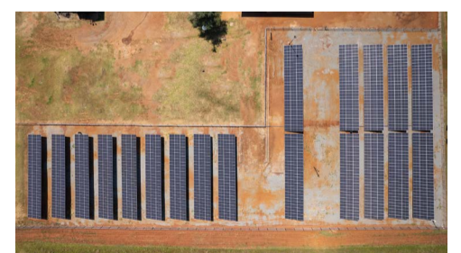
Almost a hectare of photovoltaic panels – supported by lithium batteries for seamless continuity – generates around 726 kW of power.
