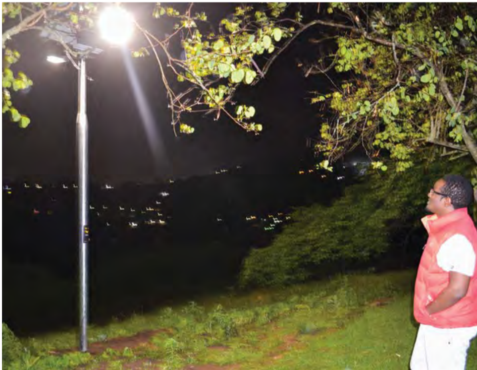
Six solar-powered LED lighting units were donated to the community, providing much needed lighting at night.
