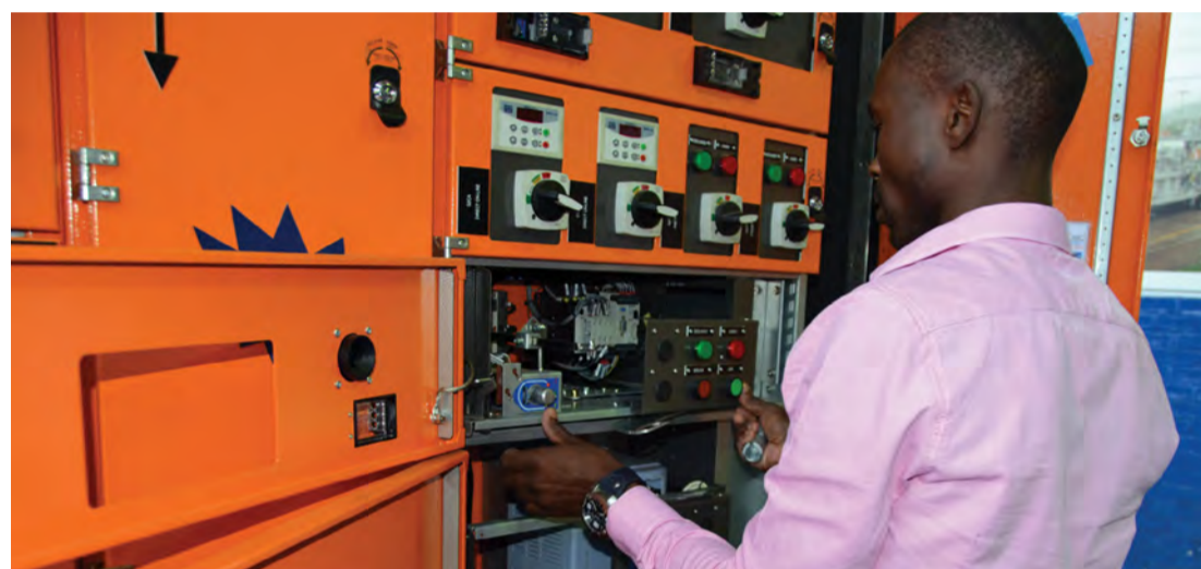
A fully withdrawable direct online starter bucket produced at WEG Automation Africa.
