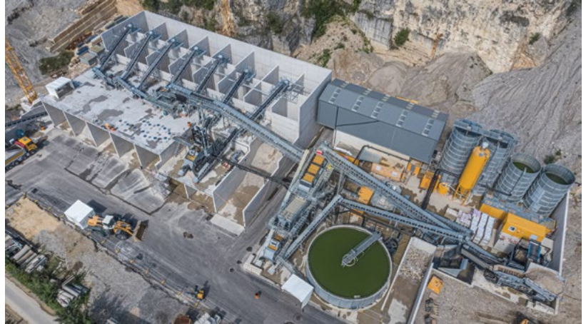
Terex Washing Systems installed a full 'Feeder to Filterpress' solution at Albin Borer, which achieves throughputs of 250 tonnes per hour of C&D and excavation waste, producing nine saleable products.
