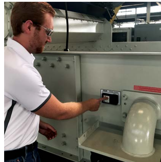
The impact test – also known as the hammer test or bump test – is now part of the company’s quality assurance programme during factory testing as well as on-site.
