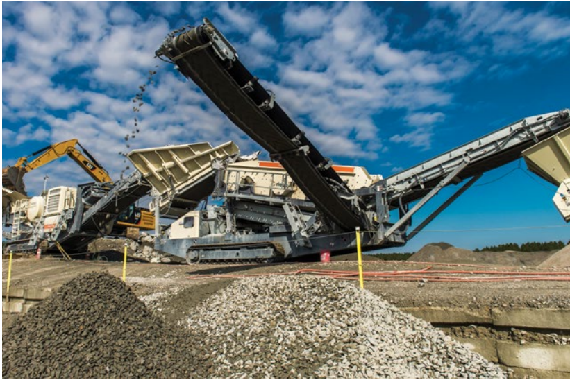
Metso mobile jaw crusher and scalping screen working on-site.
