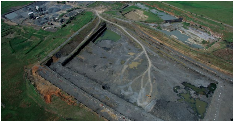
The square nature of the pit allows for particularly big blasts, which translates into massive cost savings.
