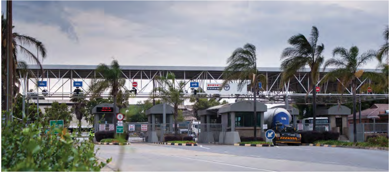
PPC's Jupiter cement plant in Germiston, Gauteng, South Africa.
