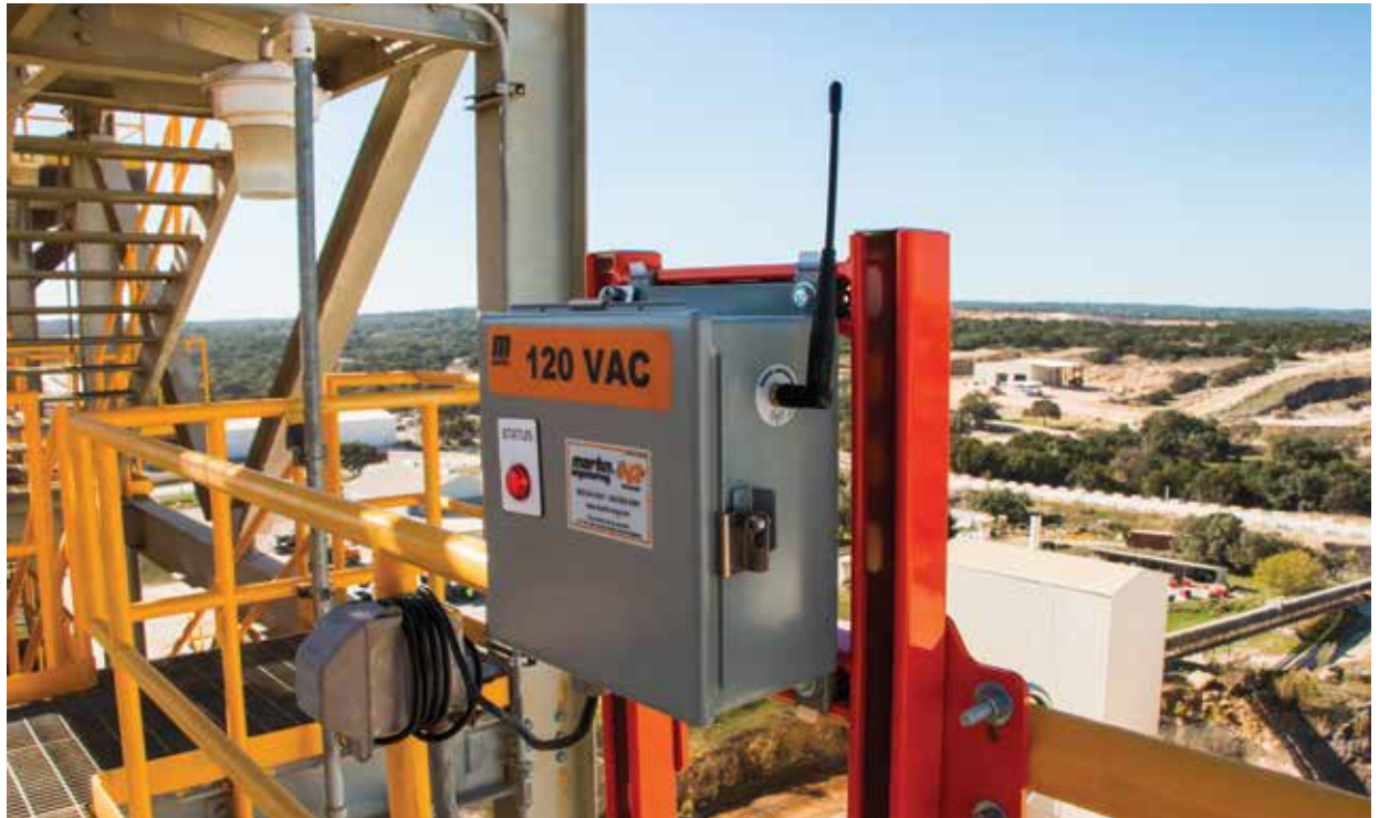
Up to 50 units can be monitored by a single gateway connecting to the Internet.
