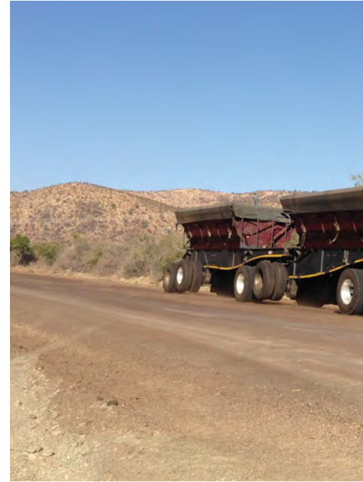
Road after treatment with FlowCentric Mining's Roadtech.
