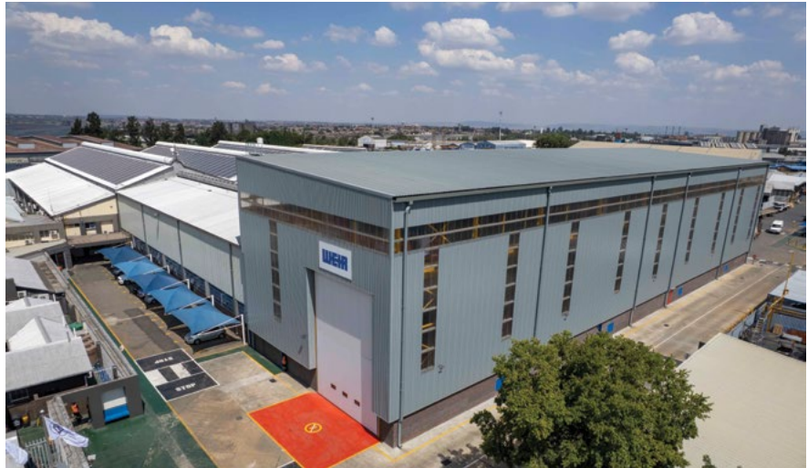
The recent expansion at Weir Alrode, which included the addition of a heavy bay screen manufacturing facility, has added a further 1 600 m 2 of dedicated production space under roof.
