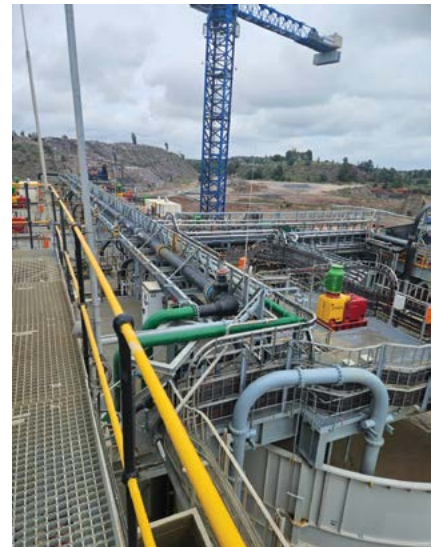
Finalizing all trades for cold-commissioning.
