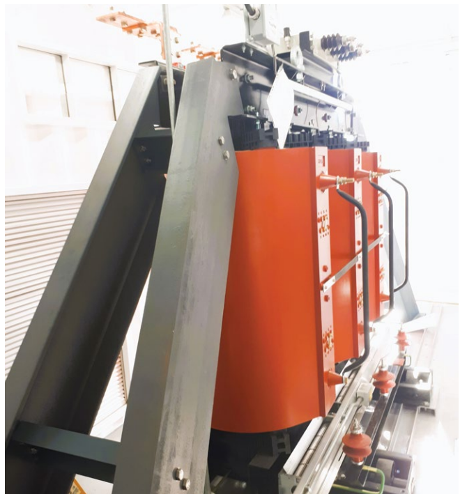
Dry-type transformers in a containerised solution for a mining application.
