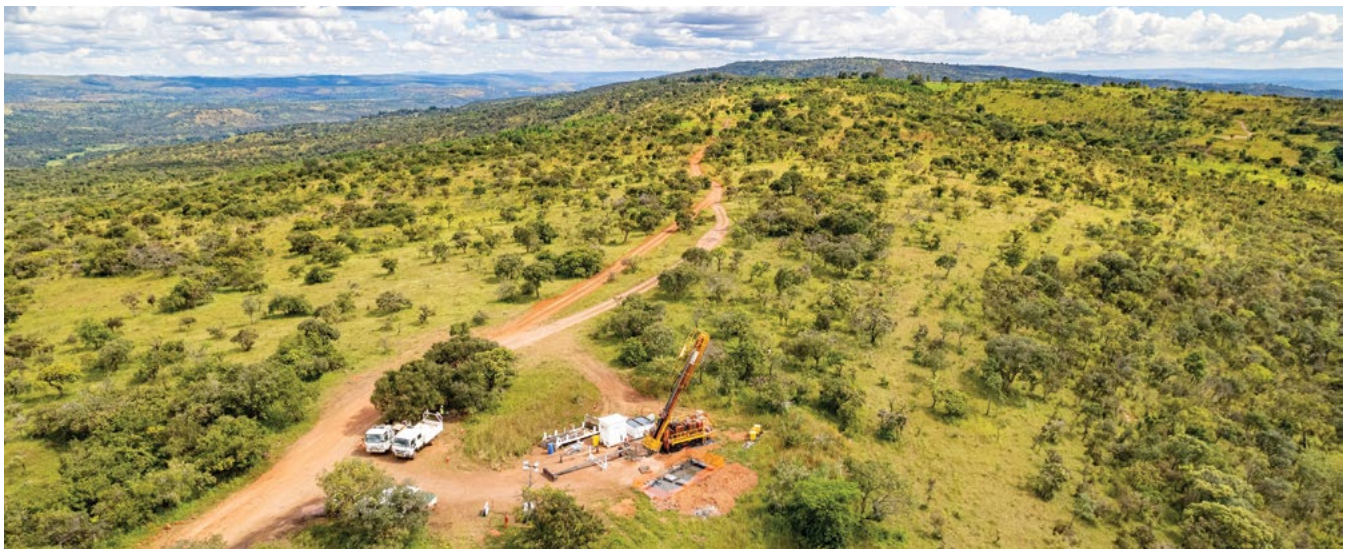
A recent Feasibility Study outlined a mine plan for 52.2 million tonnes of ore to be processed over an 18-year life-of-mine.
