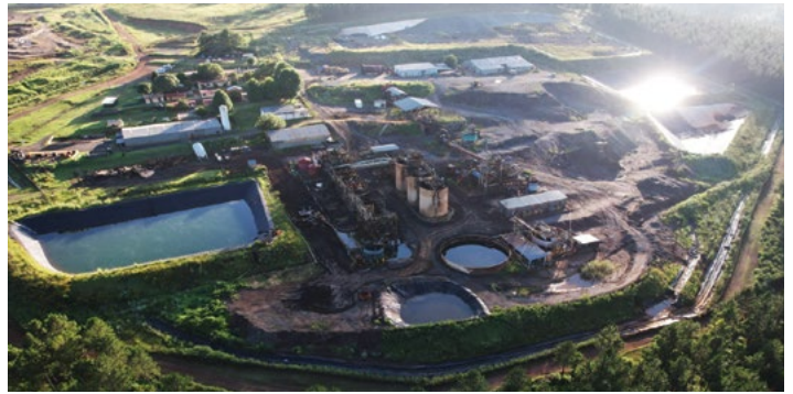
TGM is accelerating the TGME gold plant build.
