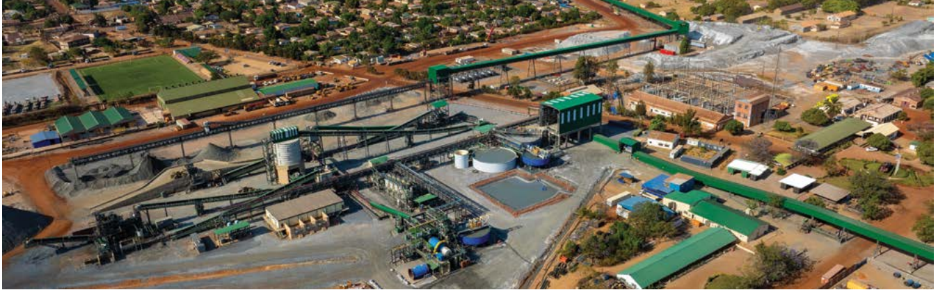
METC managed the restart of Kipushi Zinc Mine process operations from FS to commissioning. The project was completed within a tight 20-month schedule despite logistical challenges.
