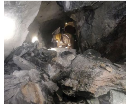
First view between the Western and Eastern tunnels.
