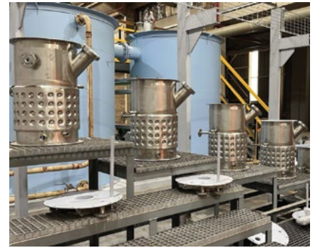
Leach reactor installation.
