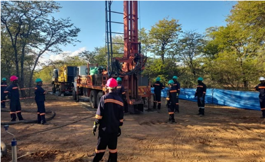
Drilling taking place at Letlhakane.
