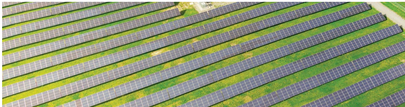
Field of PV panels for solar energy generation.
