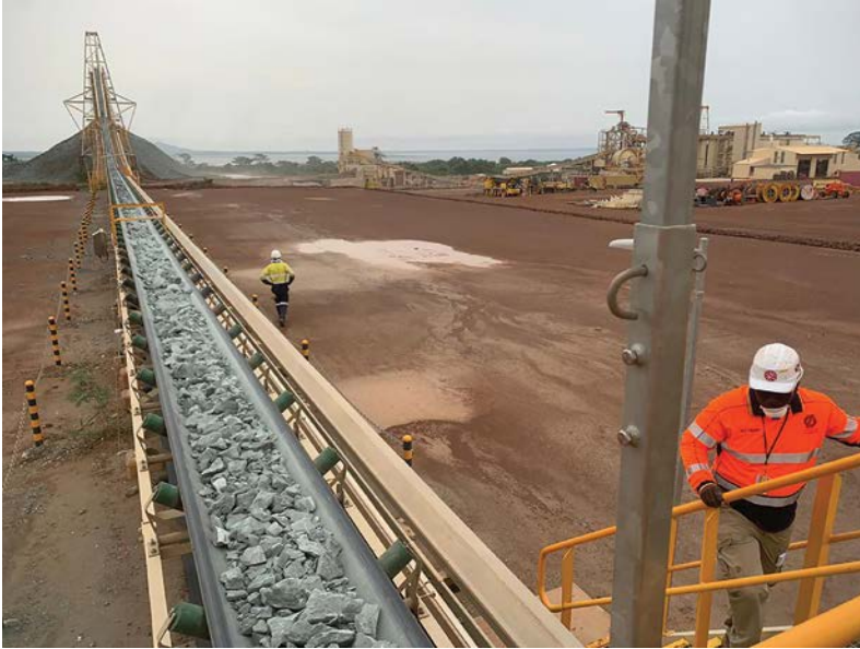
Tru-Trac's trained conveyor specialists conduct systematic conveyor inspections as part of the company's full service offering.
