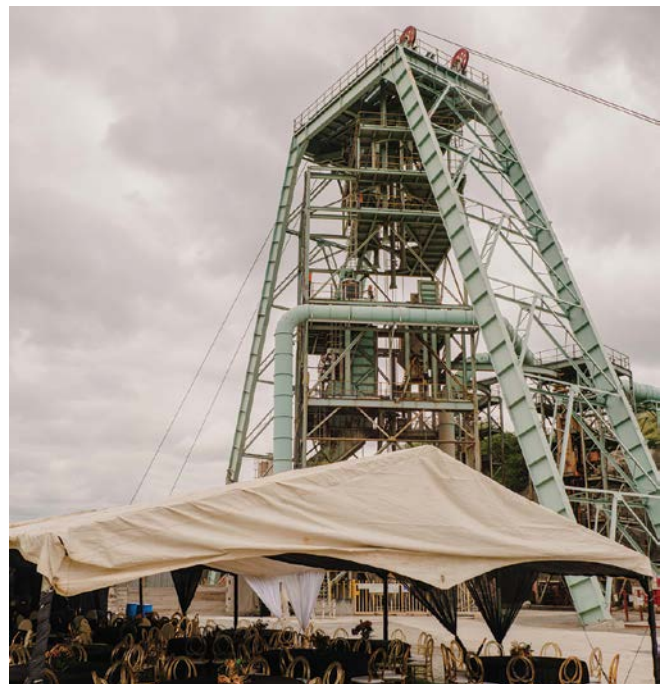
Reaching a final depth of 1 200 metres on 9 January 2024, the new ventilation shaft sunk by Murray & Roberts Cementation at Palabora Mining Company is a triumph in many respects.
