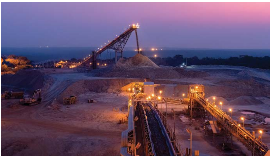
The Lumwana processing facility.
