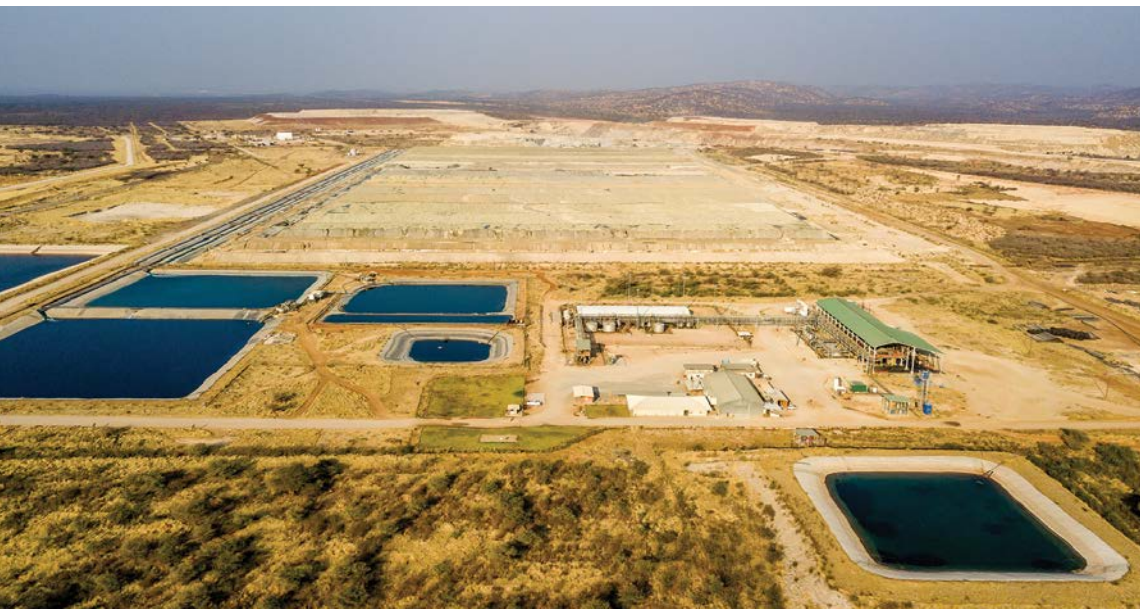
Residual Heap leach at the SX and EW plants.
