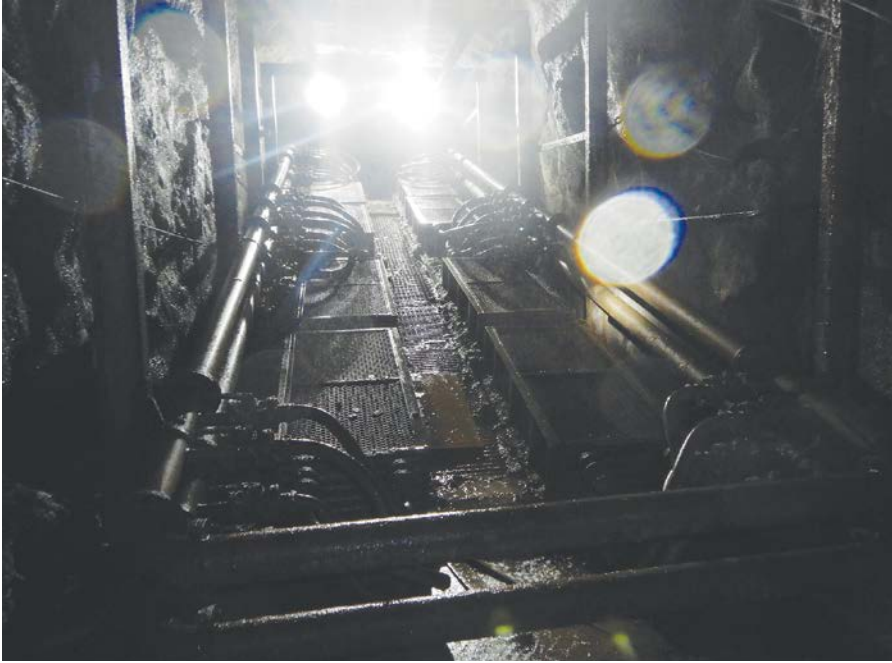
Closed-circuit cooling coils that were replaced with the BAC.
