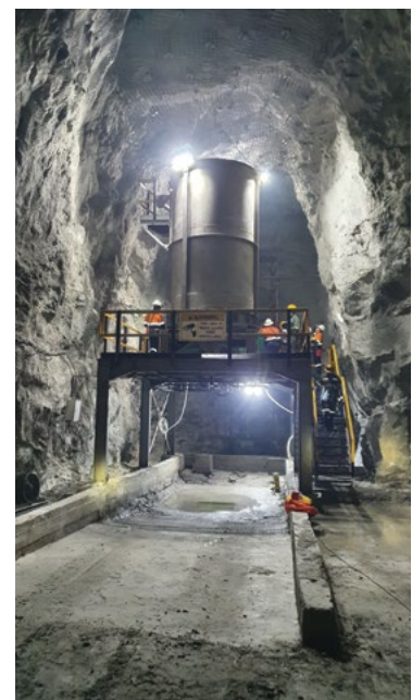
Delivering explosives to record breaking depths.
