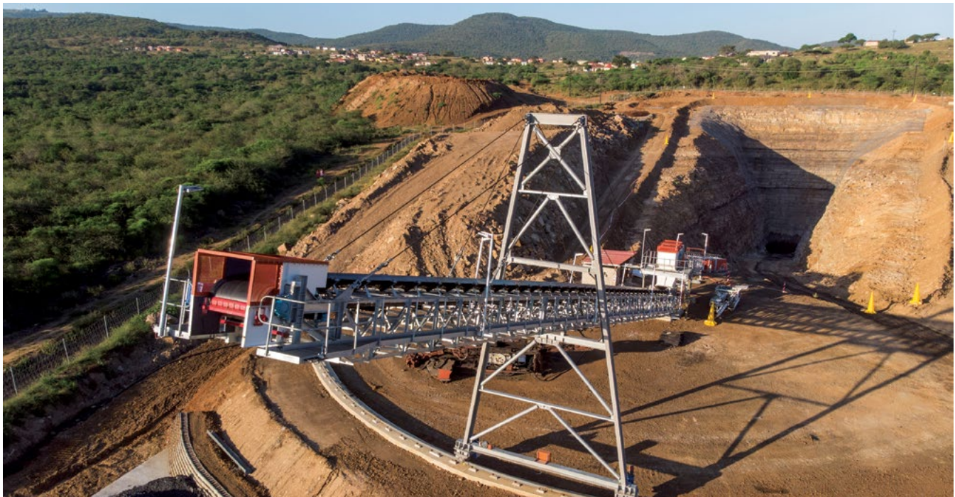
Mngeni Shaft is ZAC's newly developed shaft aimed at supporting production levels.
