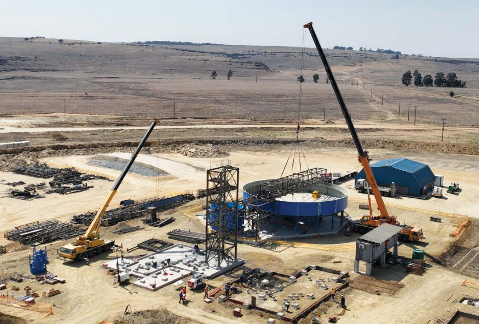
The construction of the processing plant at the Gugulethu Colliery.
