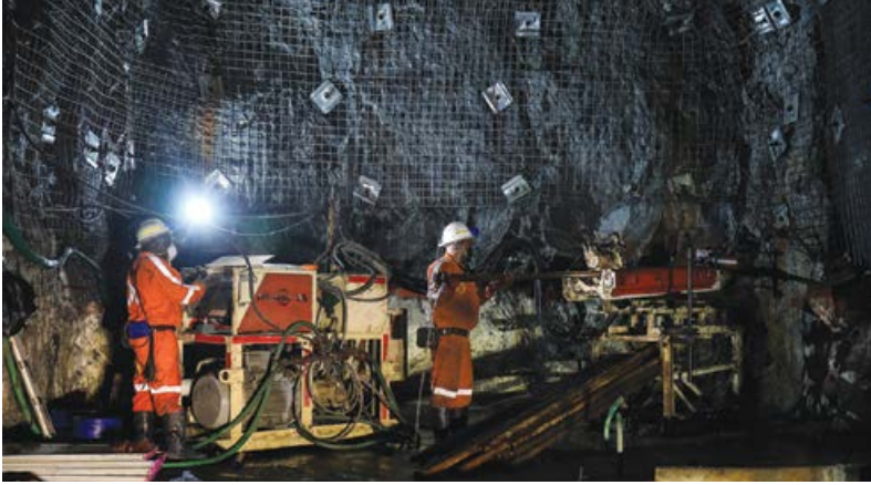
Underground drilling at Venetia Underground Project.
