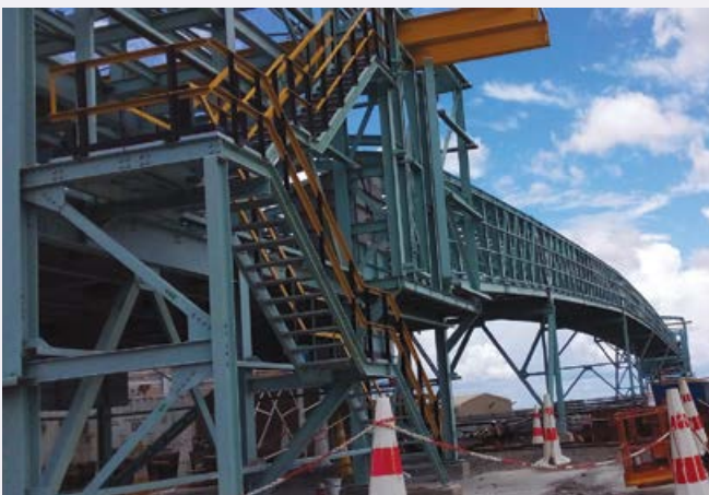
Louwill Lefa built and erected gantries for the VUP project.
