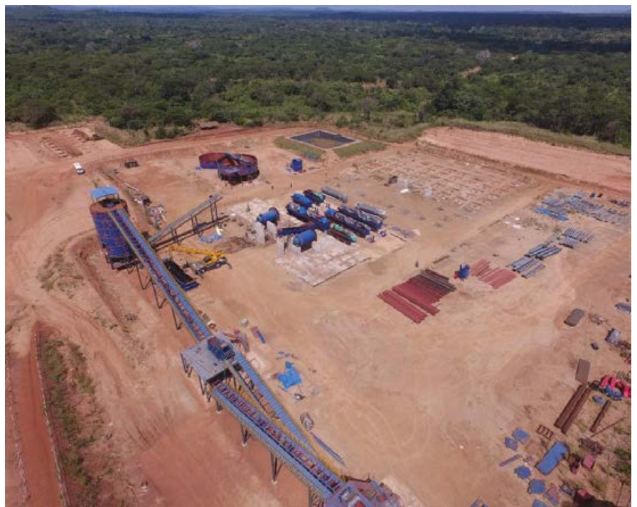
Construction on the Lindi Jumbo project is nearing completion.
