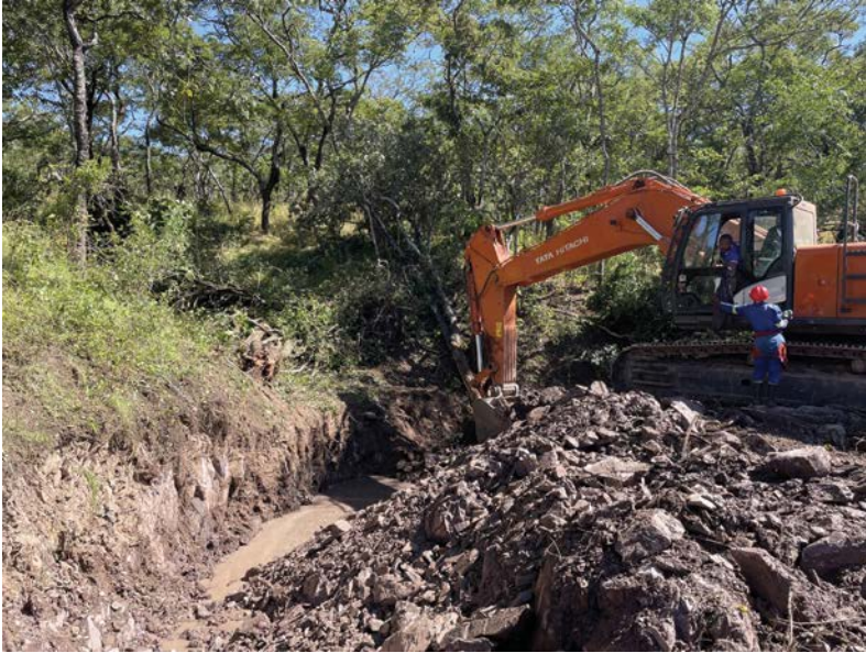
Site clearing and infrastructure development underway.
