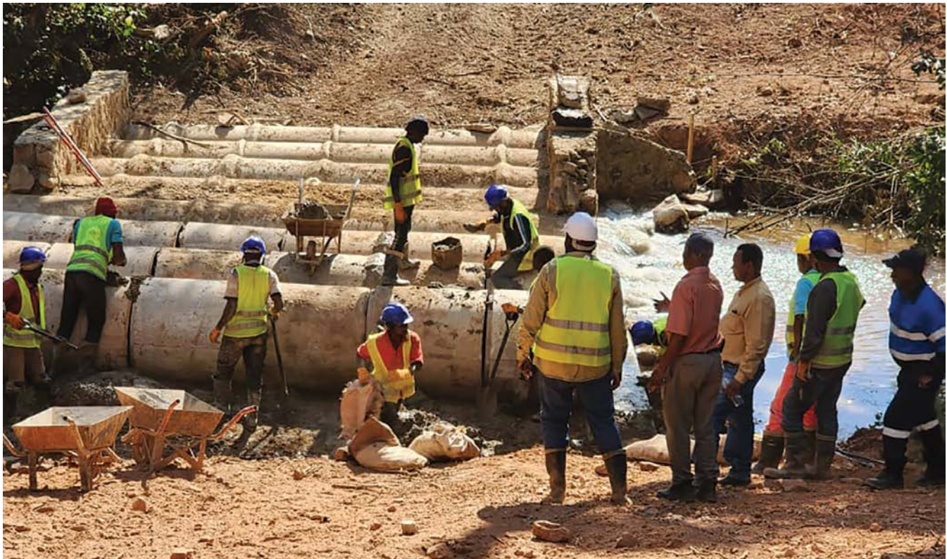
Bridge development underway at the Molulu Project.
