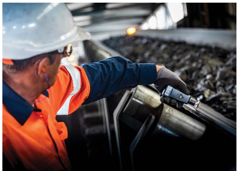
A technical advisor from Weba Chute Systems measures belt speed to ensure optimal material flow and minimal impact on the transfer chute.
