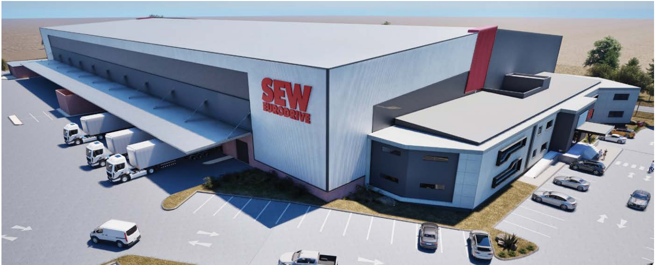
This facility will be the cornerstone of SEW-EURODRIVE's strategy to 'close the loop' by offering comprehensive repair services within Africa.
