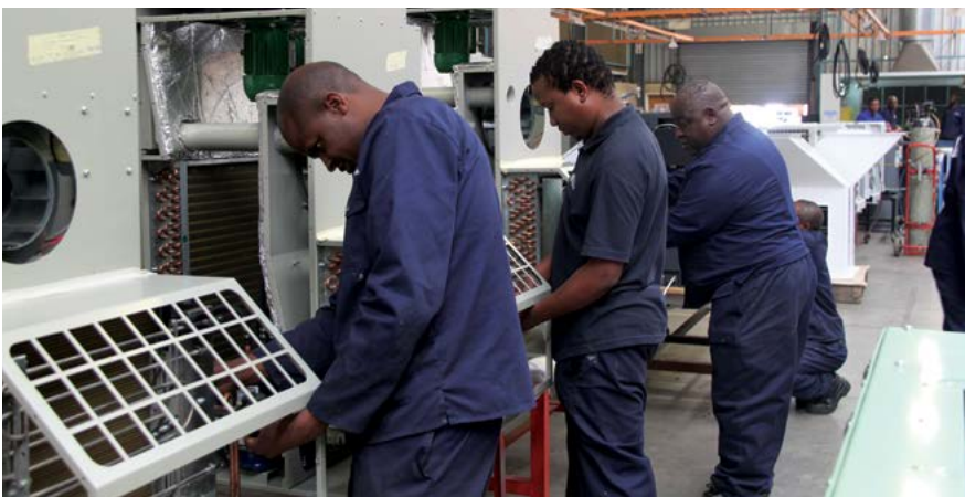
Construction of Booyco HVAC systems underway.
