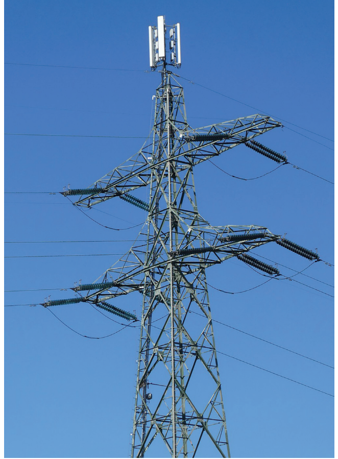
Power pylons and similar infrastructure are mostly constructed out of steel components.
