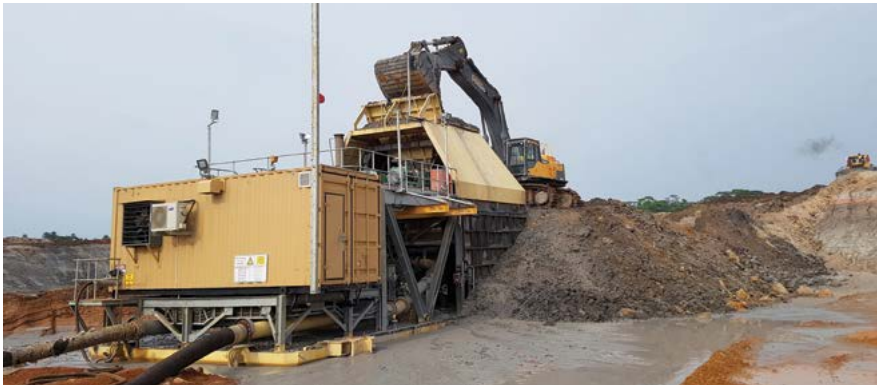
Trafo Power Solutions delivers tailored power solutions that address the unique challenges of the mining industry.
