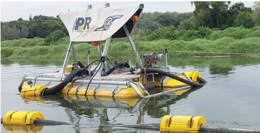
IPR's in-house designed SlurrySucker dredging unit.
