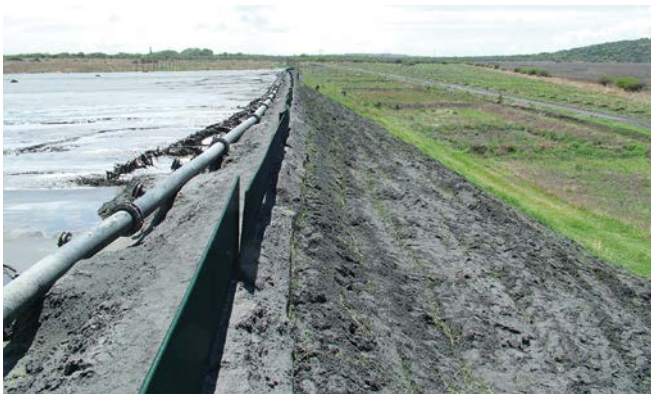
Kroondal Platinum Mine, upstream deposition with spigot system and planting of grass for erosion protection on outer side slope.
