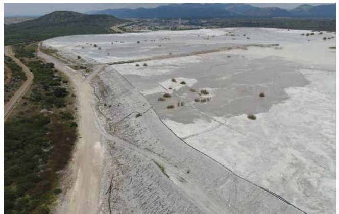
Upstream deposition with spigot system on Pilanesberg Platinum Mine.
