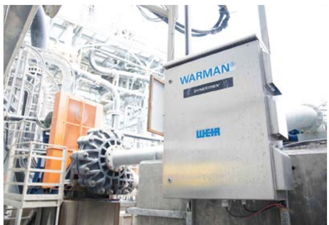
Below: A Synertrex system installed on Warman pumps at a tailings facility.
