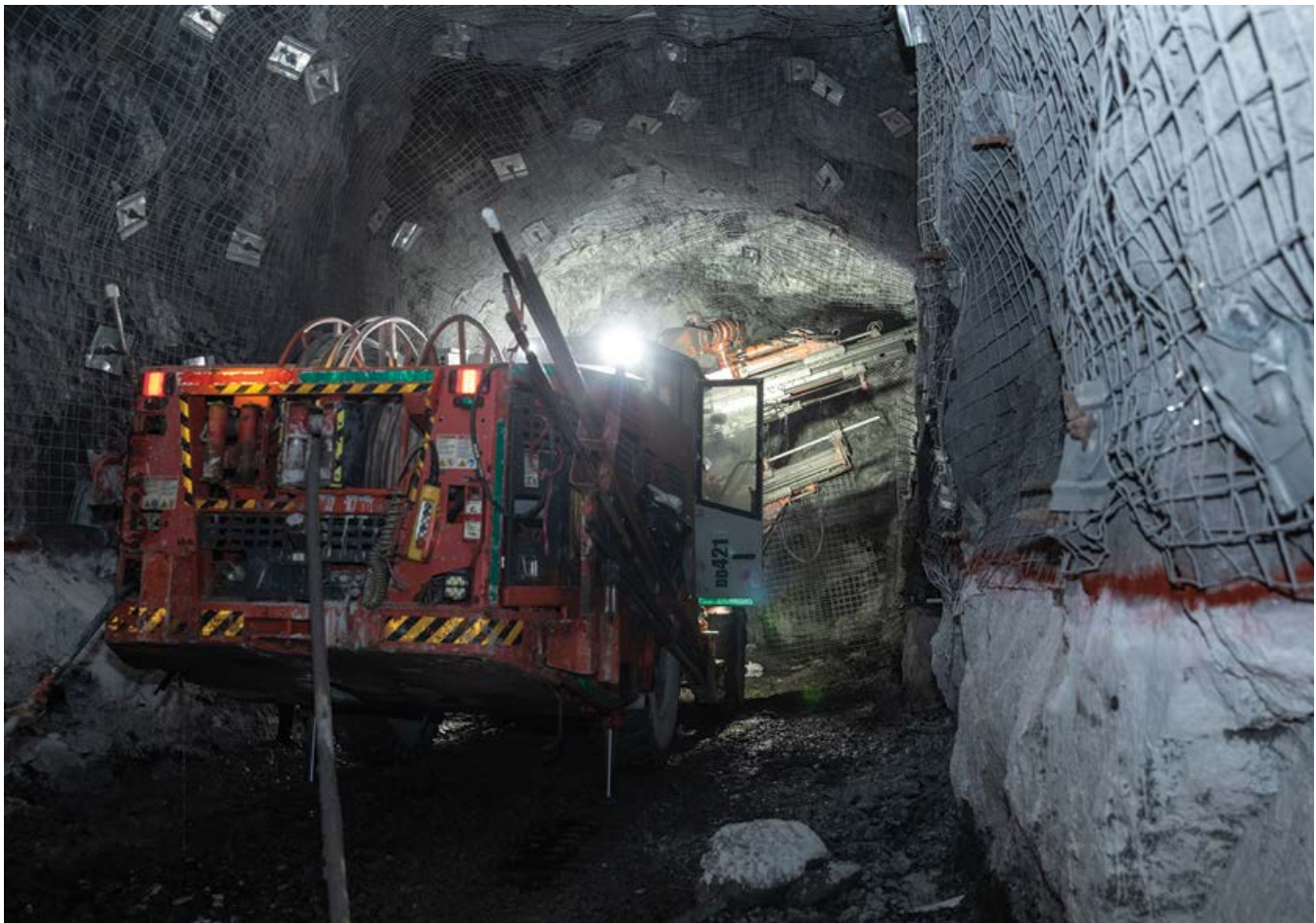
Newly developed Venetia underground mine.
