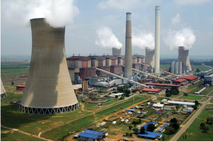
Babcock was involved in the construction of the first six units for Matla Power Station.
