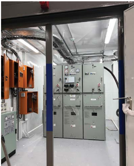
Modular substations, often referred to as E-houses, are prefabricated or modular structures that house electrical equipment and systems.
