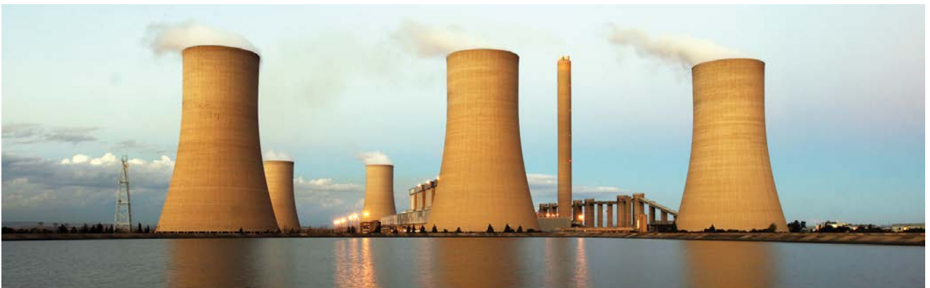
Eskom Lethabo coal fired power station.
