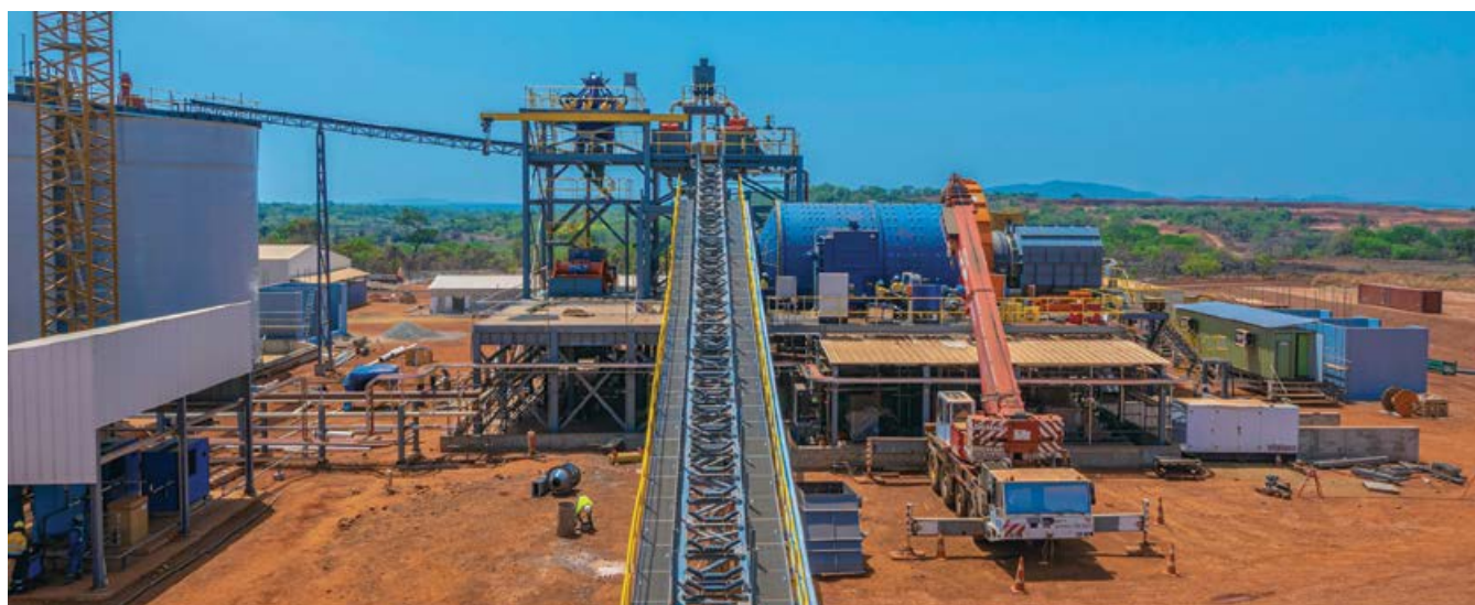
Construction of Kouroussa mine in Guinea.
