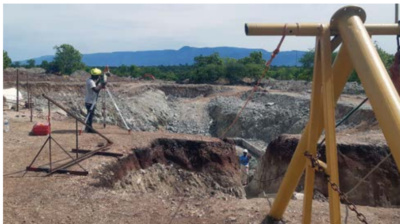
Mine development underway.
