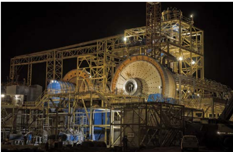
Below: T3 Projects was involved in the Essakane mill upgrade project.
