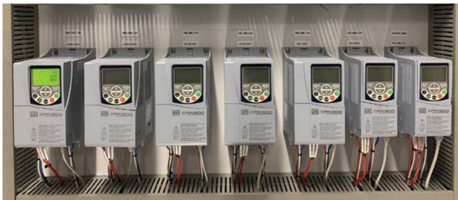
A range of WEG Variable Speed Drives that can prevent equipment from tripping out during load shedding.
