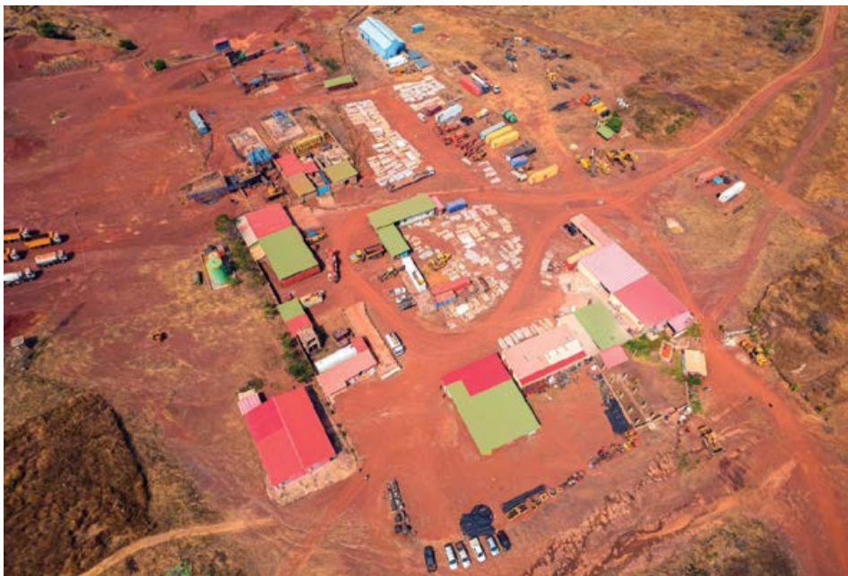
Hummingbird begins commissioning Kouroussa Gold Mine.
