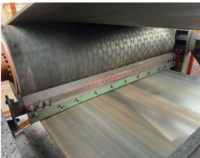
A Brelko Nip Guard installed at Grootegeluk Coal Mine.
