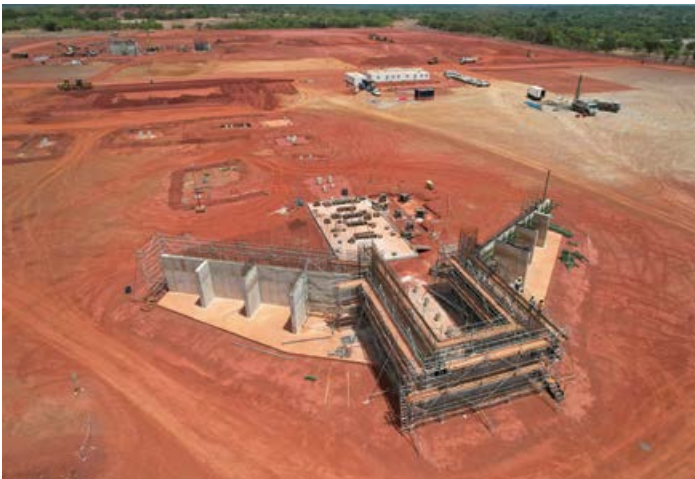
Below: Construction of the primary crushing facility.
