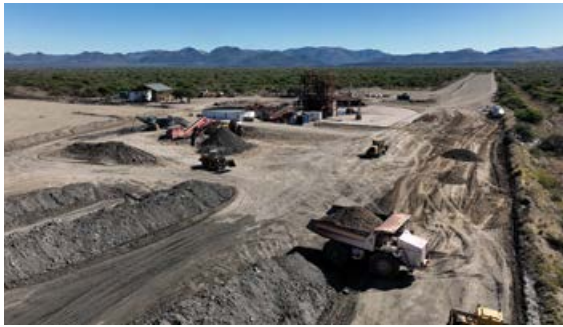
Mantengu Mining has commissioned the first of three chrome processing plants.
