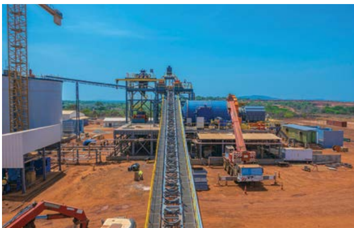
Kouroussa gold mine in Guinea begins hot commissioning phase.
