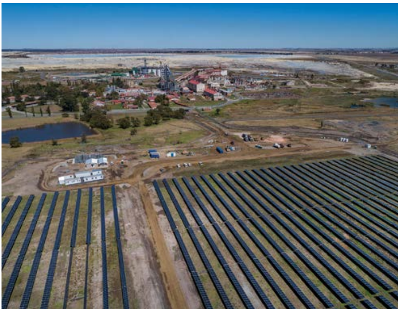
Evander solar plant with Twin Shaft 7 and 7a and Elikhulu plant in the background.
