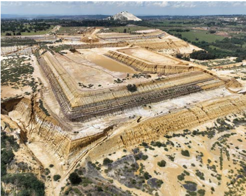
The 1L 23-25 surface dams that Pan African Resources will re-mine and process.
