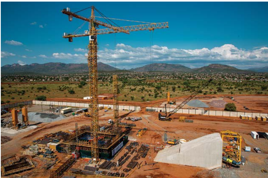
Below: Civil construction activities and preparations for Shaft 2 sinking are well underway.
