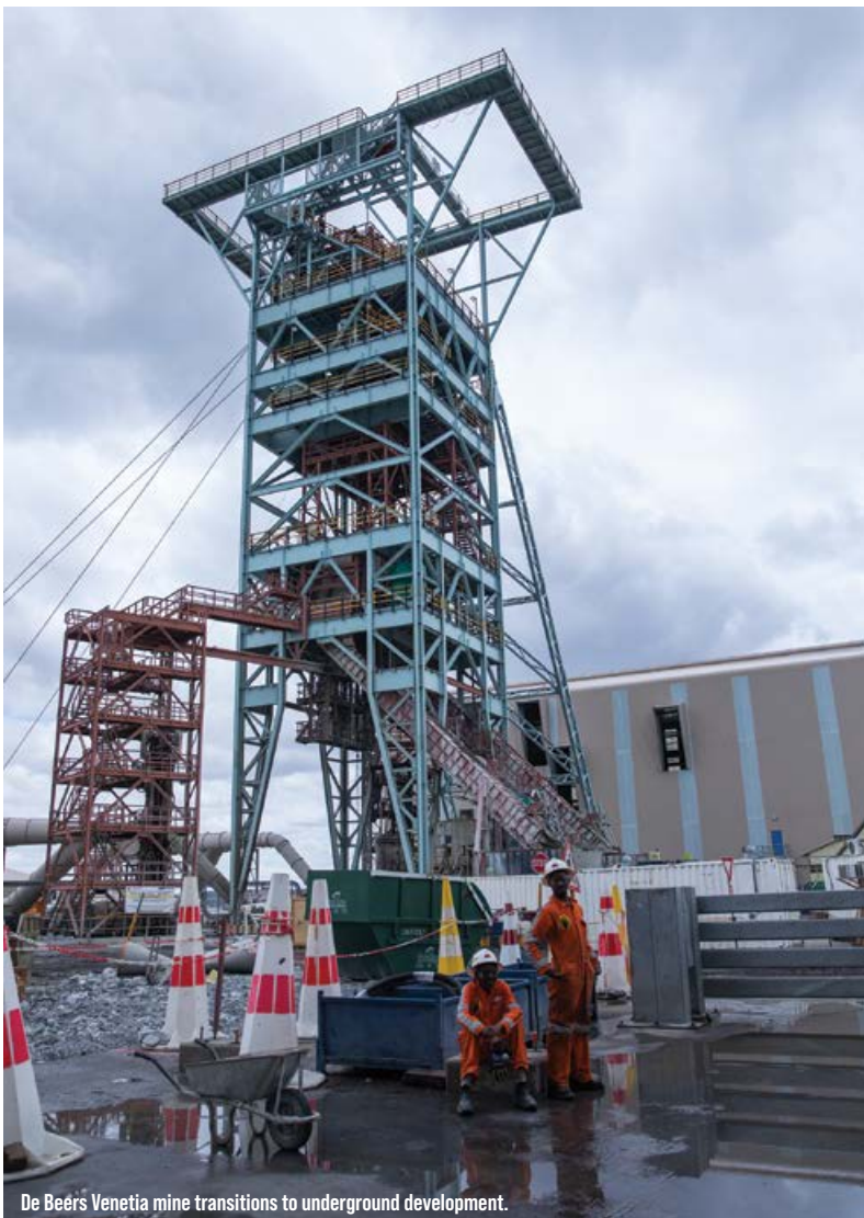
The $2,1-billion VUP is a standout project.
