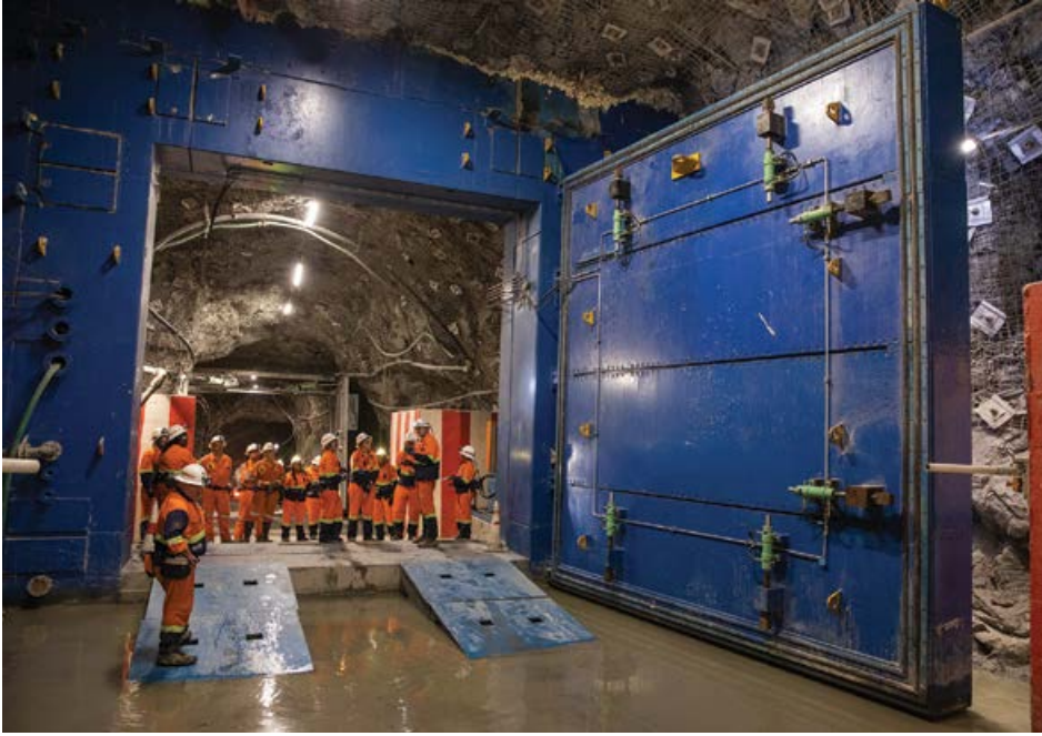
Above: The first of five water doors being installed at VUP.
