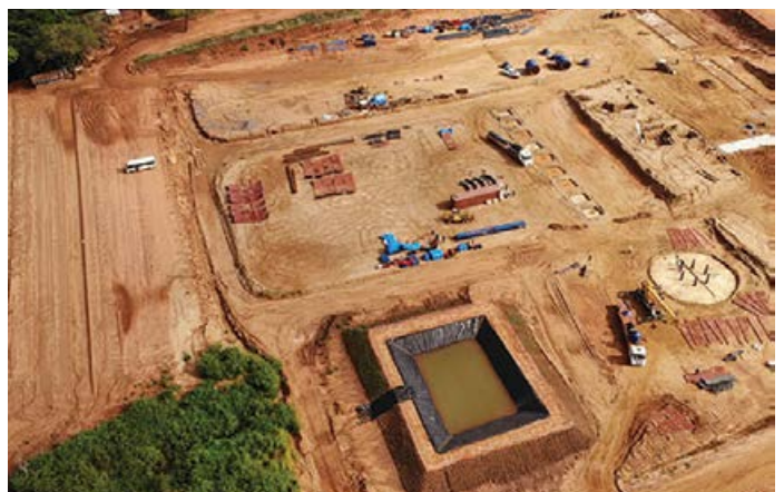
Lindi Jumbo prepares for mine commissioning.
