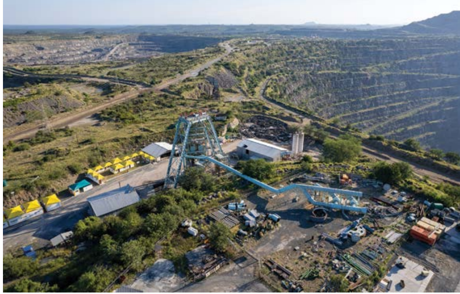
Above: A view showing the location of the ventilation shaft project at PMC.
