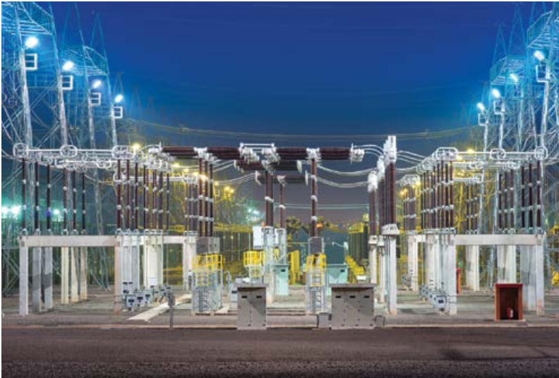
VoltVision Power helps companies reduce their static power and CO 2 emissions by up to 10%. VV Net Zero allows you to measure these CO 2 reductions accurately.
