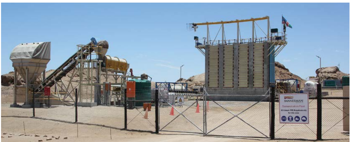
Etango Demonstration Plant.
