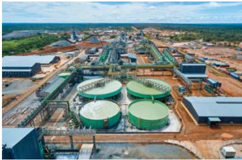
Kamoa's Phase 1 and Phase 2 concentrator plants are both in commercial production.
