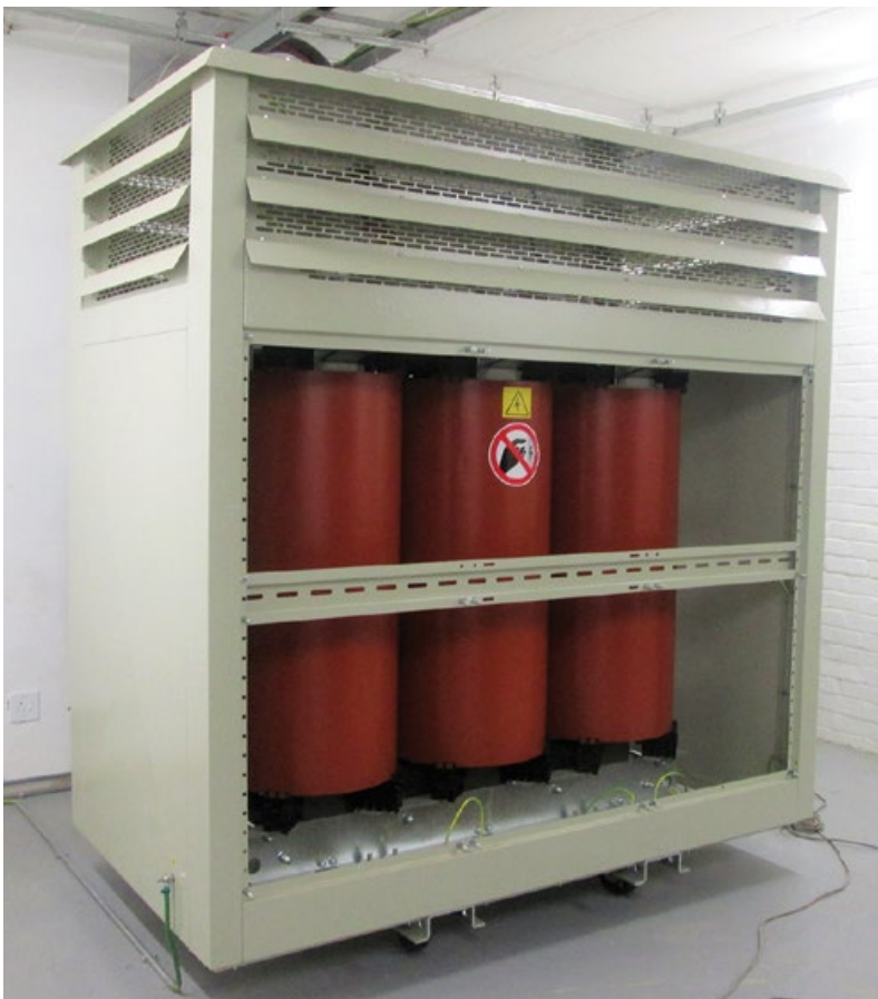
Above: Dry-type transformers provide unique advantages over the traditional liquid cooled types, including a smaller footprint and lower maintenance costs. Below: A 1800 kVA dry-type transformer designed and built to order in an IP23 enclosure.
