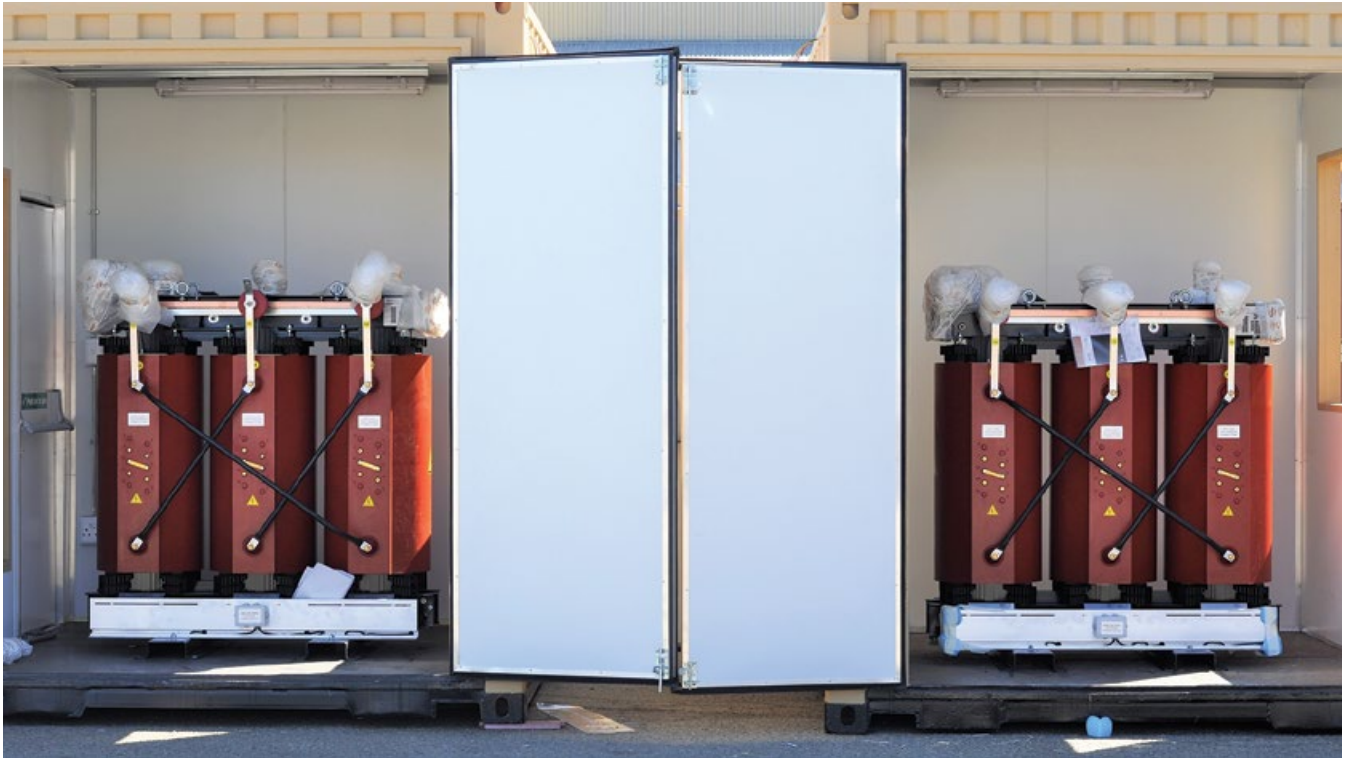
Above: Dry-type transformers provide unique advantages over the traditional liquid cooled types, including a smaller footprint and lower maintenance costs. Below: A 1800 kVA dry-type transformer designed and built to order in an IP23 enclosure.
