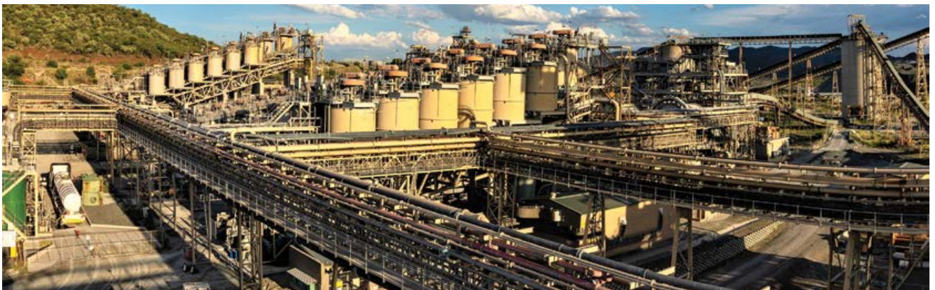
PPM Process Plant.
