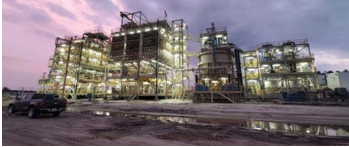
Stark Resources partners to deliver chemical free fine mineral separation.
