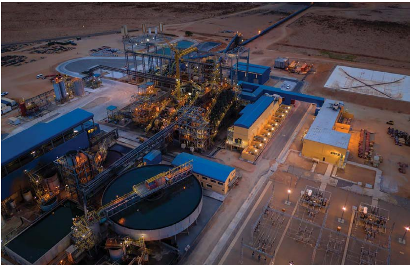
The Gamsberg project is equipped with modern infrastructure.
