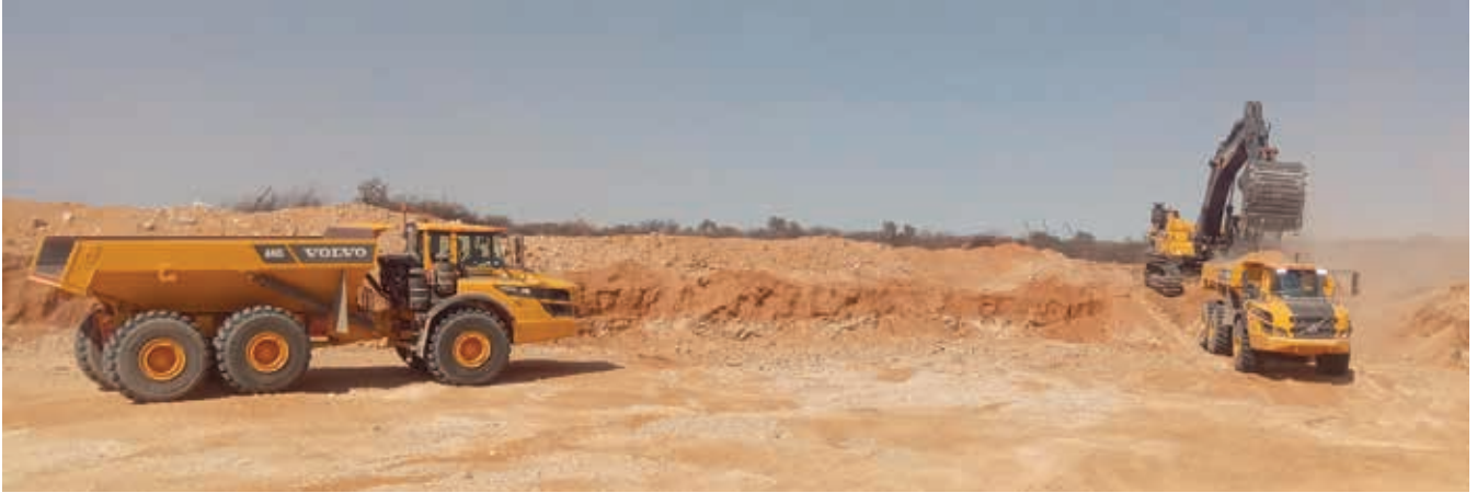
The first box cut was opened on 4 September 2020.
