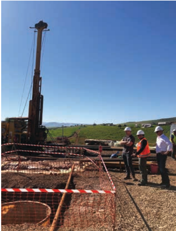
Drilling work at Emmerson Plc's Khemisset potash project in Morocco.
