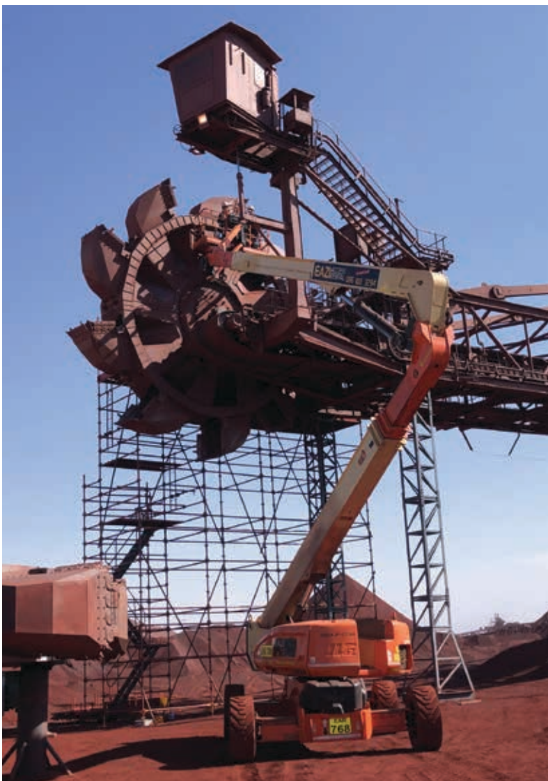
New cylinder installation during a bucket-wheel replacement project.
