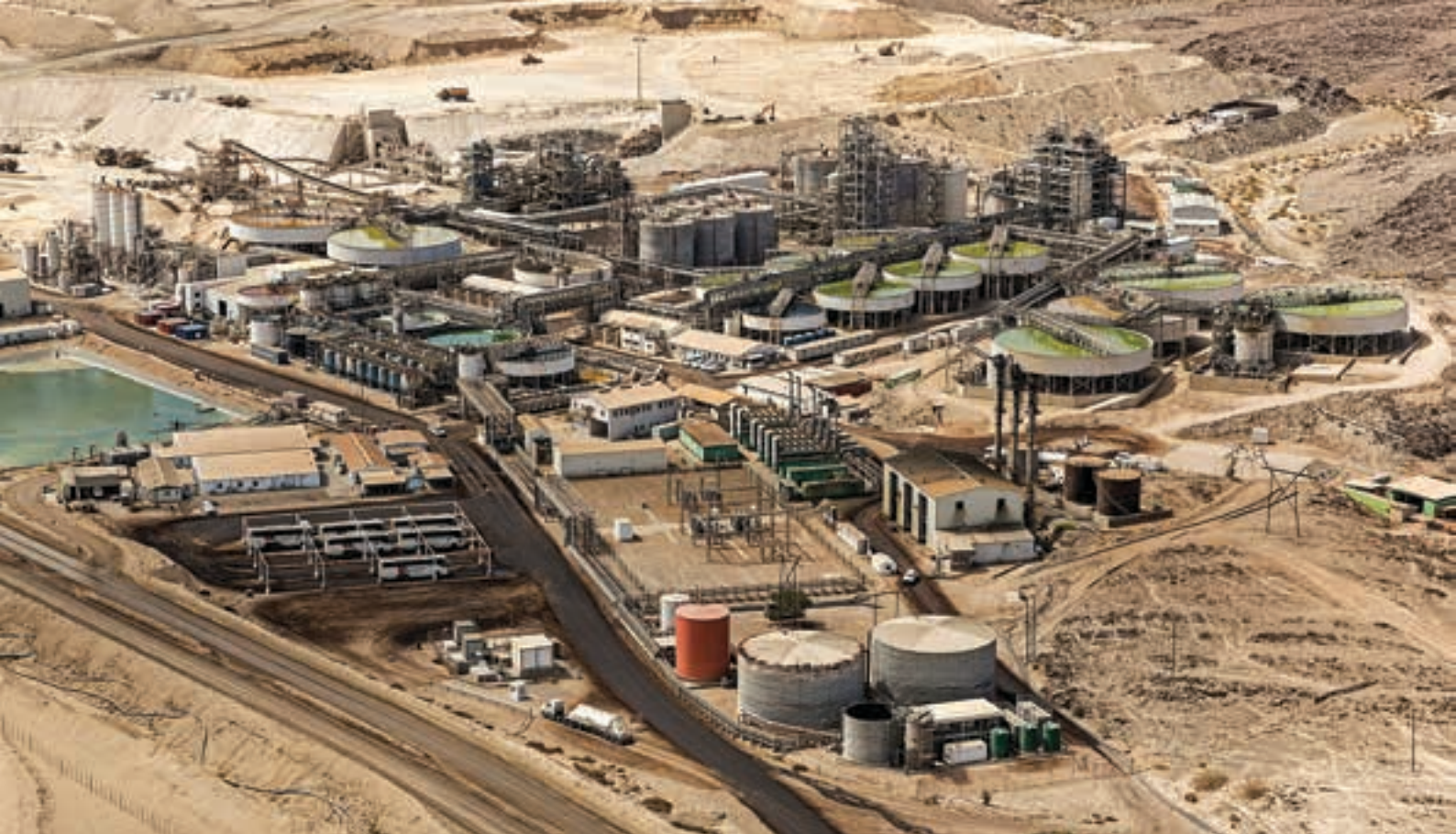
Aerial photo of Langer Heinrich Mine taken in March 2018 (photo: Paladin).
