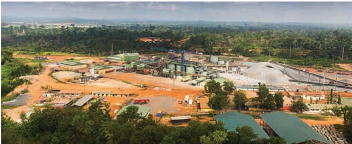
View of the Asanko Gold Mine (AGM) in Ghana (photo: Asanko).
