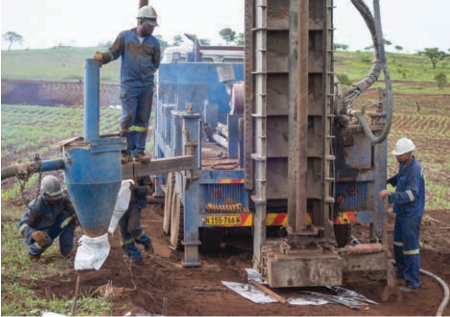
Reverse circulation drill rig at work in November 2019.
