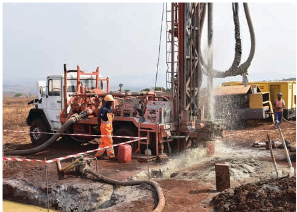
Waterbore drilling at Longonjo in September 2019.
