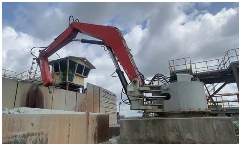
Left: Installation of the refurbished Sandvik BR3288i hydraulic breaker and BB8094R breaker boom has been completed, and the unit is now ready for testing in the primary crushing circuit. Right: Coupling of the main boom to the pedestal is underway as part of the Sandvik rock breaker installation.
