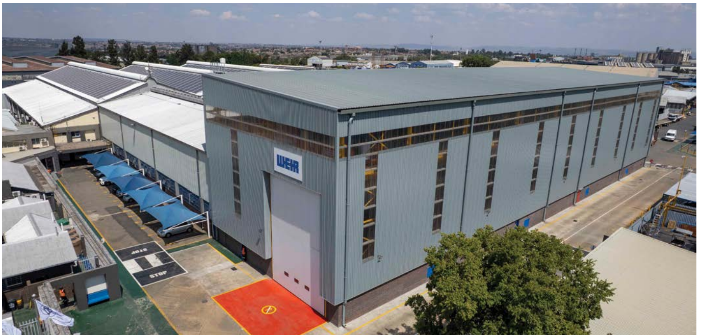
The recent expansion at Weir Alrode, which included the addition of a heavy bay screen manufacturing facility, has added a further 1,600 m 2 of dedicated production space under roof.
