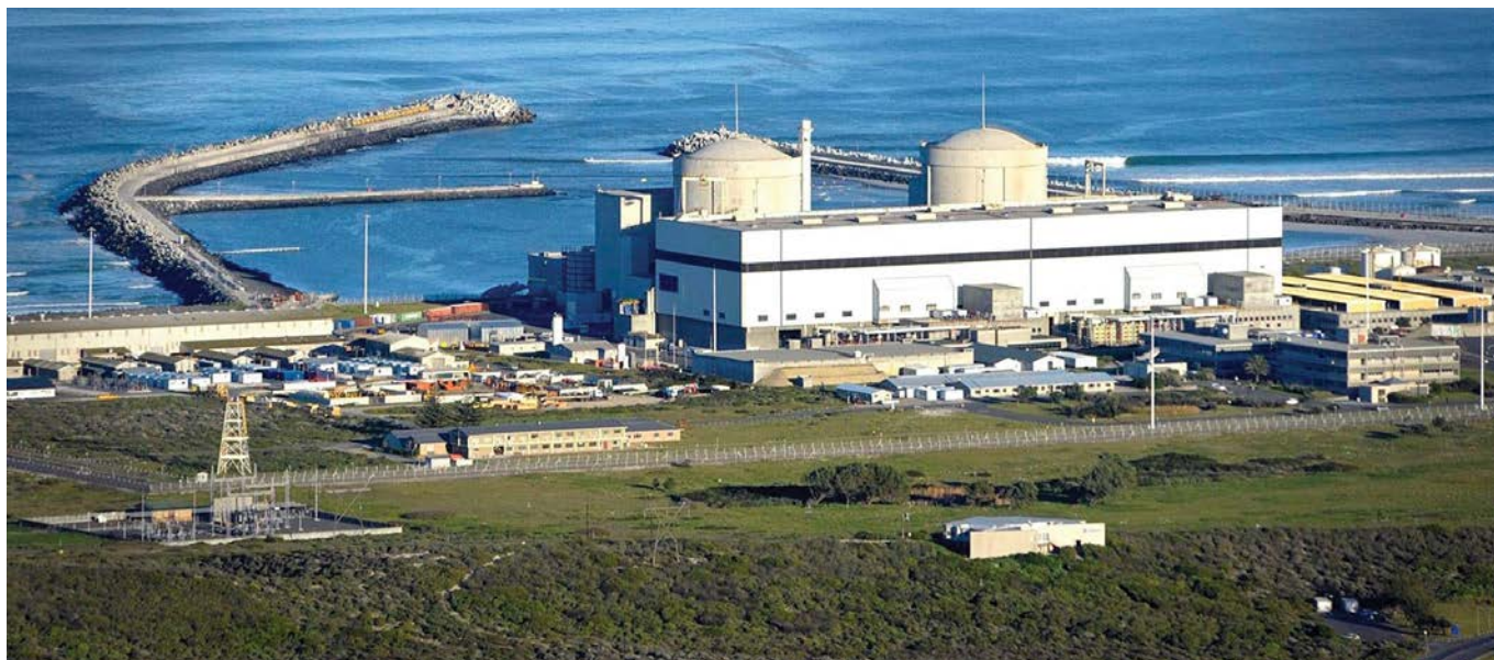
The two-unit Koeberg Nuclear Power Station with a capacity of approximately 1 854 MW is currently the only nuclear power plant on the African continent.
