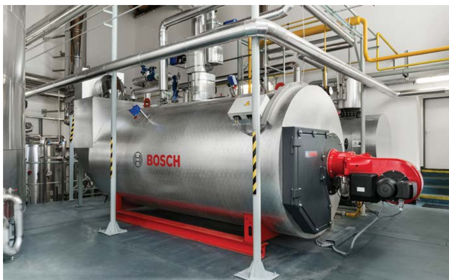
By replacing a 30-year-old boiler with a new Bosch UL-S steam boiler, a brewery in the Czech Republic improved operational reliability and reduced fuel costs by approximately 16%.
