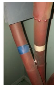
Left: A PD graph on medium voltage (MV) terminations trended over time. The escalation in Q_{max} (mV) as the resistance of the insulation deteriorates is evident until failure occurs, which trips the supply voltage. Right: Typical partial discharge (PD) failures owing to inadequate clearance between the unscreened areas of the cable termination. PD causes the build-up of a white acid-type powder due to the ionisation of the air around the activity.
