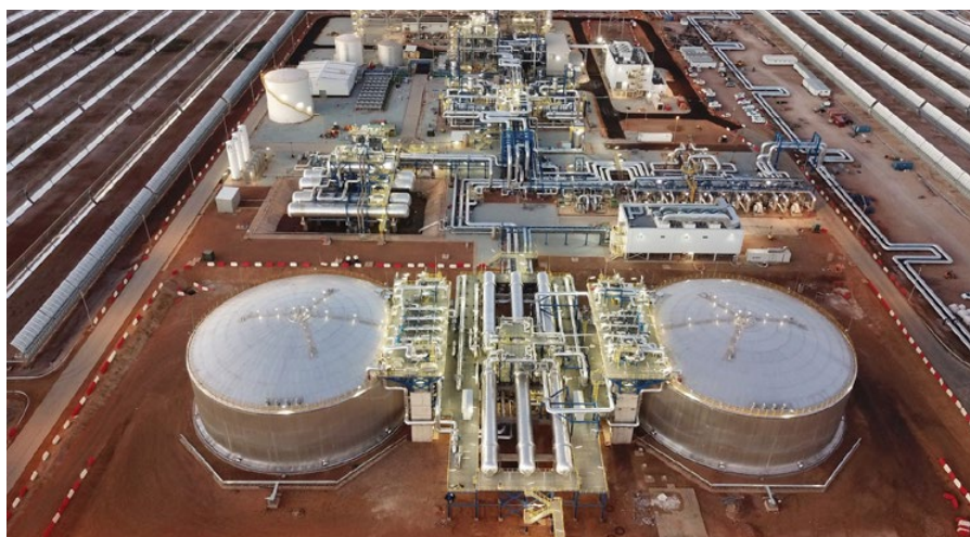
The Kathu Solar Park in the Northern Cape, which is a dispatchable CSP IPP project with a combined generation and storage capacity of 100 MW. With the lifting of the embedded generation threshold to 100 MW, self-generating operations of this size become possible, with the electricity able to be 'wheeled' through the transmission grid, subject to wheeling charges and connection agreements with Eskom and relevant municipalities.
