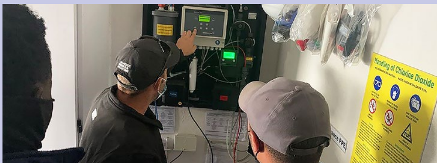
Operators conduct inspection and checking reports to ensure optimal performance, and that proportional dosing flow is maintained.
