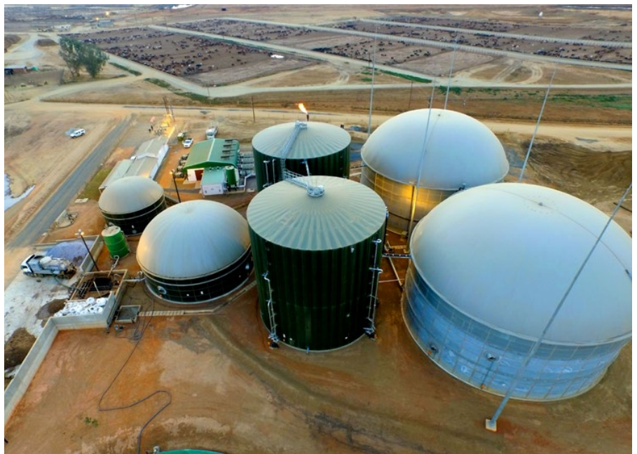
The Bronkhorstspruit Biogas Plant.
