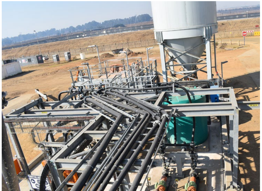
A view from the top of Nafasi's lime slaker plant showcasing the water tank, Grundfos booster pumps, calcium hydroxide storage unit and reactor.
