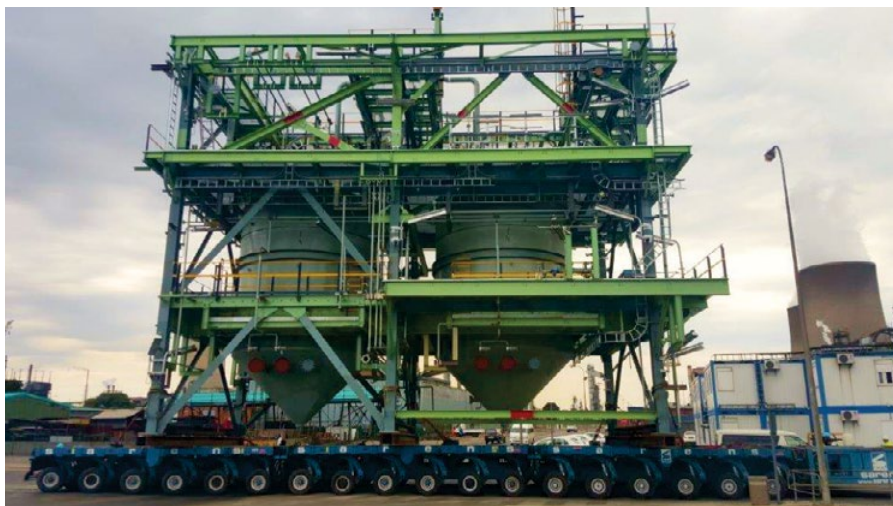
Modular plant has to be purpose designed with structural integrity so it can be safely and easily transported, placed and connected-up onsite in a ‘plug-and-play’ manner.
