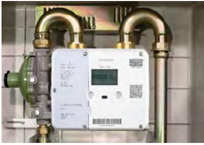
Mesura's PRODIGI ultrasonic smart meters from Energas are mainly used for large-scale housing developments.
