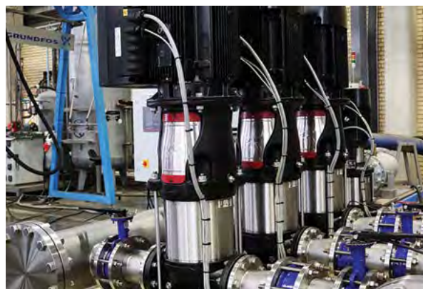
Left: Grundfos XL CR systems combine hydraulic efficiency with high efficiency IE3 motors making them ideal for use in water treatment plants and pressure boosting stations. Right: For high flow applications, Grundfos can also supply large multiple pump solutions of up to six pumps, and each pump will only run at the speed required to meet demand.
